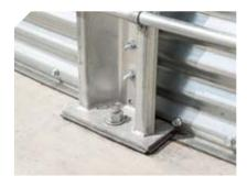
**Base stiffeners** on Ag-Comm bins are used to anchor the bin to the concrete foundation for strength, stability and bin integrity.
