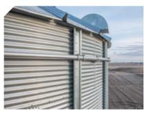
Wind rings are standard on larger sizes and optional on others and can be easily mounted to the stiffeners. Wind rings provide improved wind load—and help maintain the round bin shape when using off center unloading such as a side draw system.
