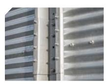
**12** gauge splice ensures that stiffeners are properly butted to effectively transfer sidewall load to the foundation.
