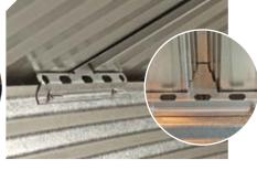
Specially designed 12-gauge eave clips connect roof sheets to sidewalls. "Up" position helps exhaust moisture-laden air. "Down" position preferred for long-term storage. Built-in rib stops keep out pesky birds. Continuous eave ring is used in lieu of clips on 54' (16.46 m) and 60' (18.28 m) models and are optional on smaller diameters.
