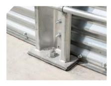
**Base stiffeners** on Ag-Comm bins are used to anchor the bin to the concrete foundation for strength, stability and bin integrity.
